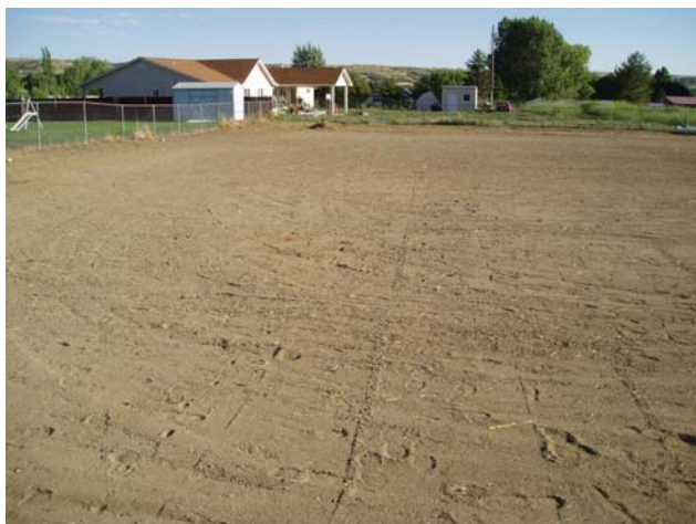
Site is graded and ready to Hydroseed
